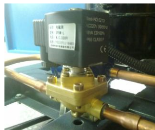
Picture 2-34: Solenoid Valve
