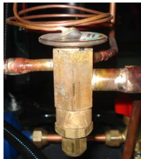
Picture 2-30: Heat Expansion Valve
