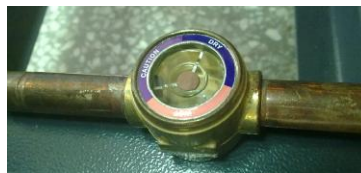
Picture 2-33: Refrigerant Indicator
