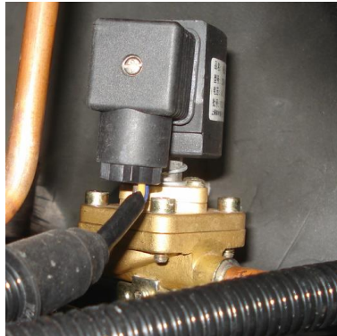
Picture 2-35: Heat By-pass Valve
