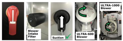
There **MUST** be a negative pressure (suction) from the blower intake. If there is positive pressure (blowing out), then the 3-phase rotation is NOT correct, and two phases must be swapped to reverse blower direction. Blower direction must be clockwise.
