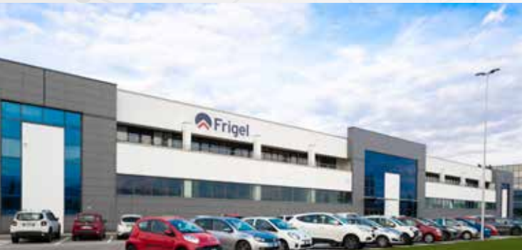
FRIGEL Firenze Headquarter Fertigung, Service, Vertrieb Firenze - Italy
